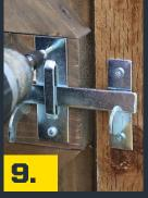
Mark the fixing holes of the jump staple and fix with screws provided.
