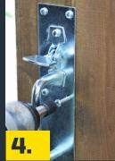
Mark the fixing holes of the thumb latch back plate, drill pilot holes and fix with screws provided.
