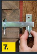
Position the keep on the post so that the latch bar sits in the notch of the keep when closed. Mark the fixing holes of the keep. drill pilot holes and fix with screws provided.
