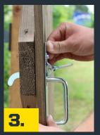
Pass the lever from the thumb latch through the slot ensuring it can be fully raised and lowered.
