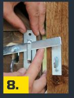
Slide the jump staple over the latch bar and position on the gate level with the keep and ensuring the latch bar can fully engage and release.
