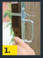
Position the latch at the required height on the gate, normally at the height of the gate cross strut.
