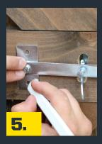
Position the latch bar on the rear of the gate style above the thumb lever so that is level when the lever is down and overlaps the gate post by at least 35mm. Mark the fixing holes of the latch bar.
