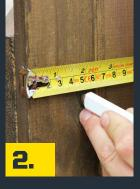
Measure 50mm from the leading edge of the gate and mark a vertical line 38mm long. Cut a 38 x 10mm slot through the gate on this line.
